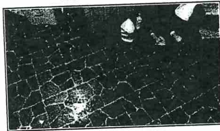
LAUNDRY AREA FLOOR
