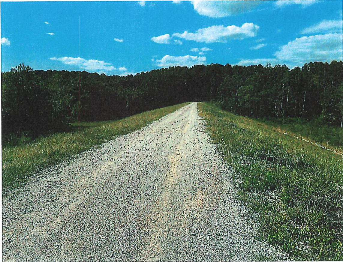
Photo 1 – Gravel-Stabilized Road on the Crest of the Tarrant Flood Mitigation Dam
