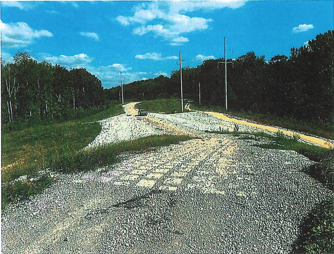
Photo 2 – Stabilized Emergency Spillway on the Tarrant Flood Mitigation Dam
